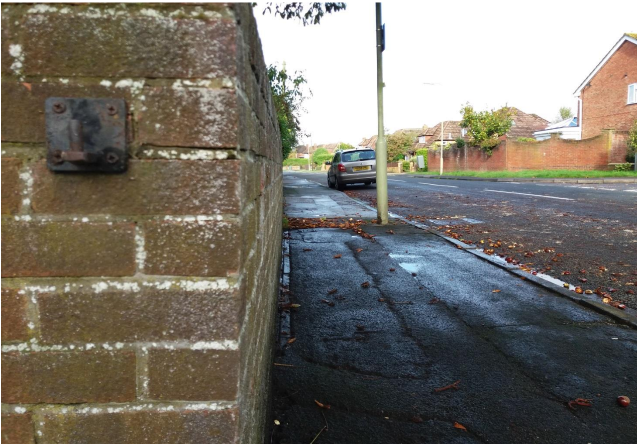
View adjacent to wall looking west
